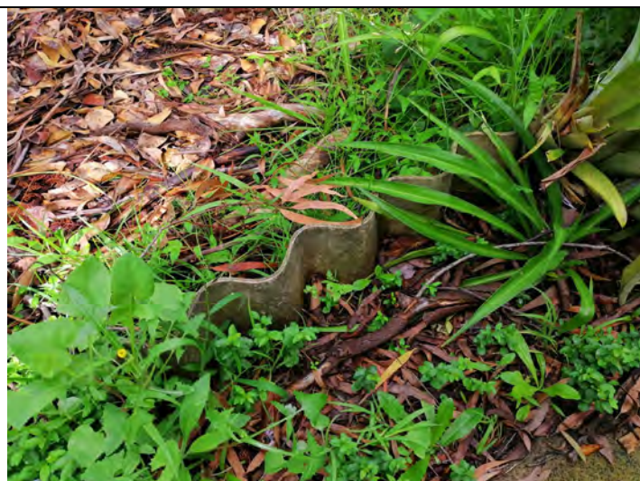
Image 3: Fibrous cement sheeting along the side pathway at 5 Canberra Ave, St Leonards.
